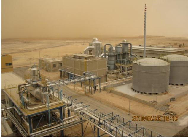
The process of powder type TSP producing is known as ROP, it is similar with normal super phosphate producing process except the acidification step that phosphoric acid makes phosphate stone more acidic. The reaction product is a powder form that can be used in secondary operation of ammonia process to produce chemical fertilizers mixtures of NP and/or NPK. TSP granular type is better and more common to use compared with powder type. ROP process involves four steps:
